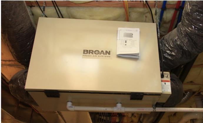
**Figure 1:** Heat Recovery Ventilator (HRV) used to provide mechanical ventilation in a residential application.
